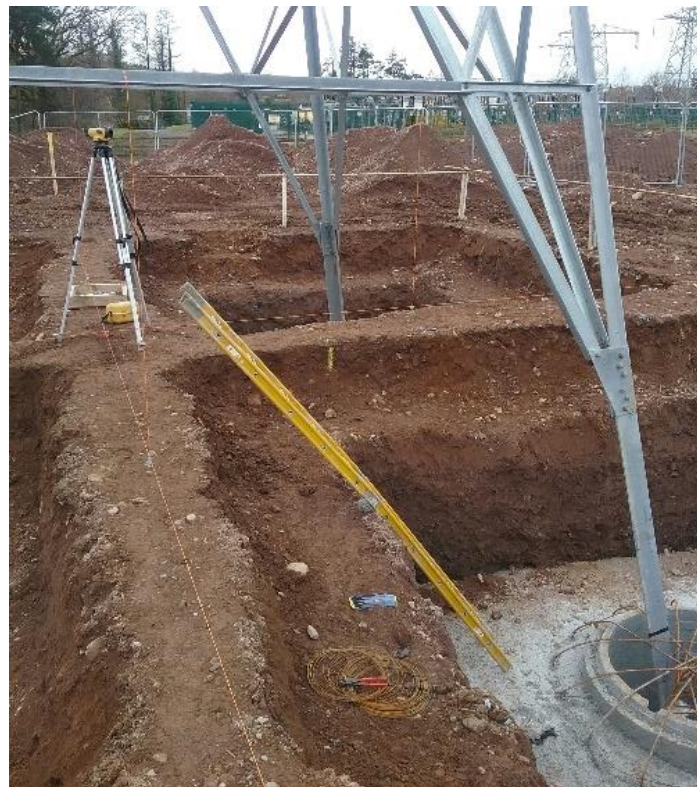
Figure 4: Typical 110kV mast foundation excavation
