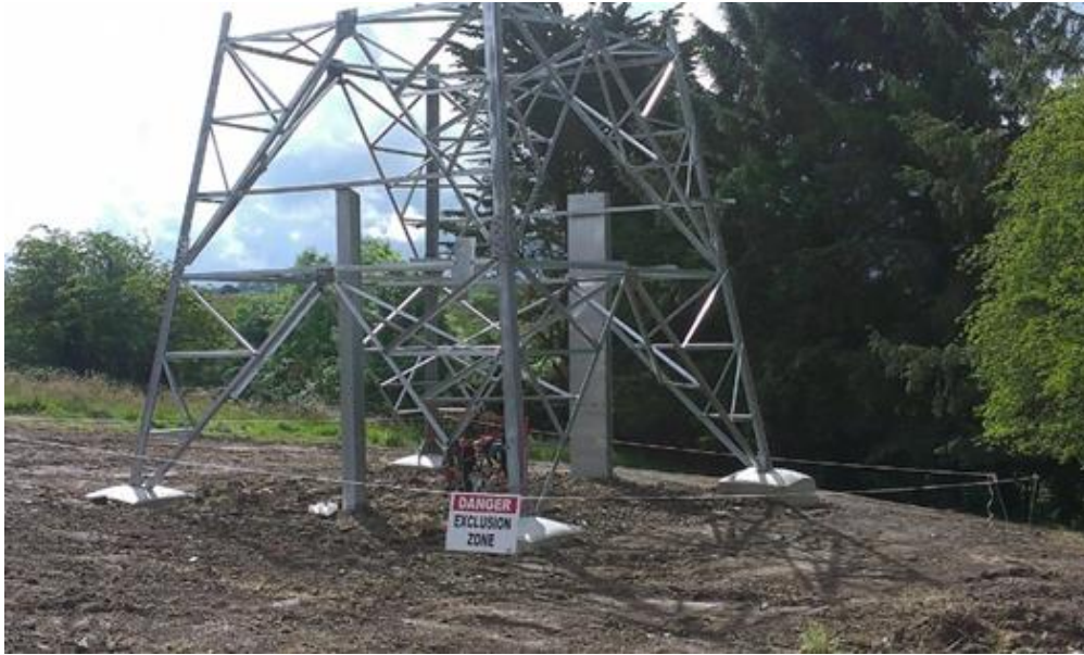
Figure 5: Base of mast structure backfilled
