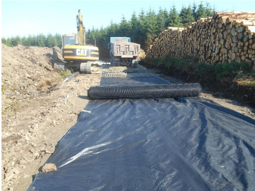
Figure 18: Crushed Rock Roadway Build-up With Geotextile
