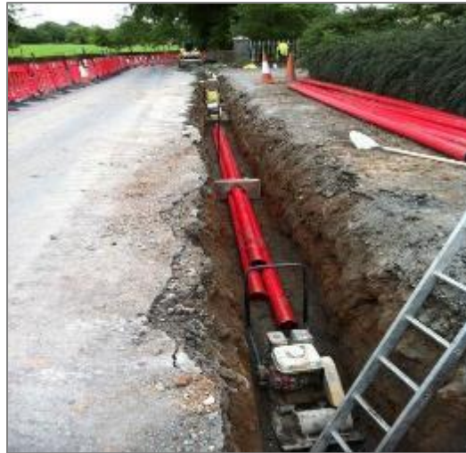
Figure 10 - Typical 110kV Underground Duct Installation
