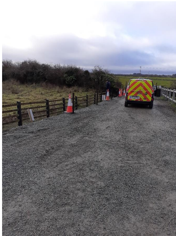
Figure 17: Crushed Rock Roadway
