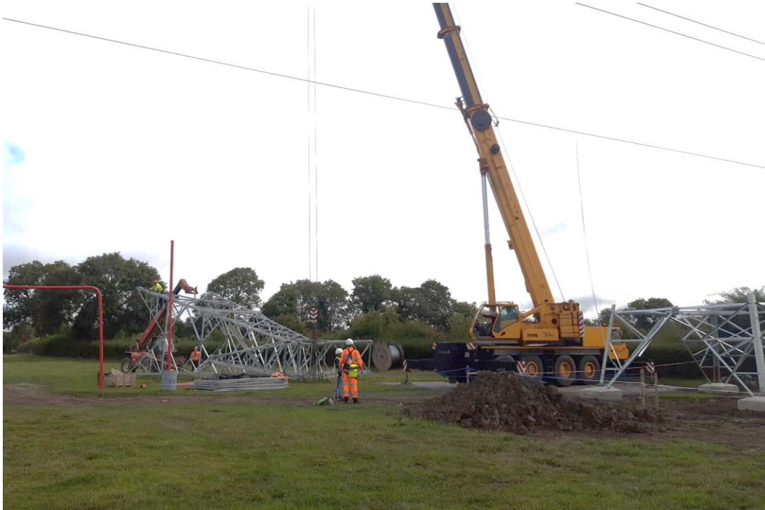
Figure 19: Crane pad and laydown areas
