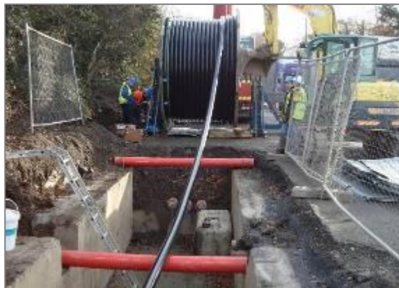
Figure 14 - HV cable pulling procedure (Typical drum set-up)
