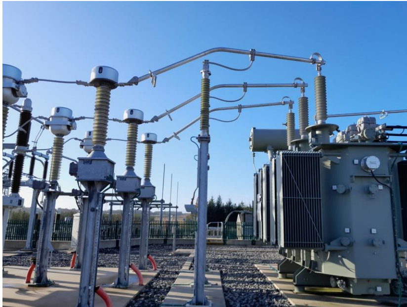
Figure 9: Typical 110kV Transformer Connection
